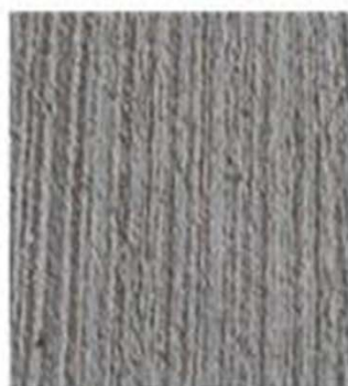
Unsealed Brushed Concrete
